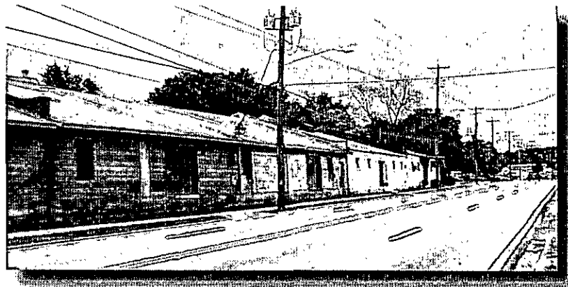
Vacant Warehouses on Gaines Street
